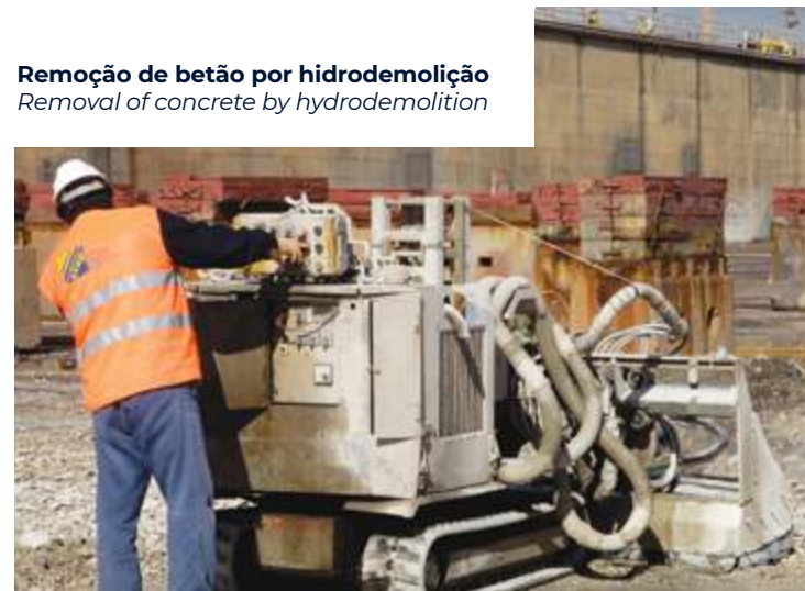
Reparação das paredes, no interior da doca 21 Repair of walls, inside Dock 21
