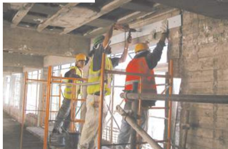
Injeção com resina de base epoxídica Injection with epoxy-based resin
