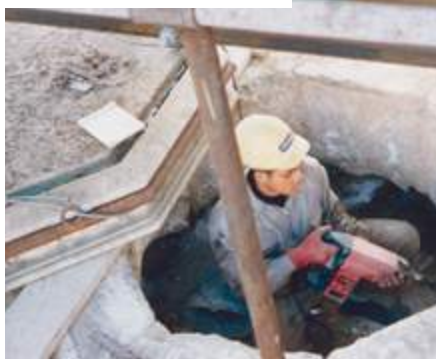
Suspensão do bronze e remoção da pedra de capeamento do pedestal Lifting the bronze statue and removal of the pedestal cover stone
