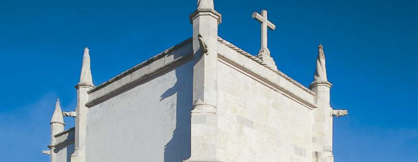
Vista da Capela durante a intervenção View of the Chapel during the work
