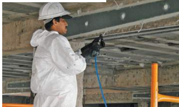
Injeção com resina de base epoxídica Injection with epoxy-based resin
