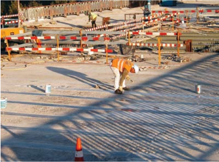
External reinforcement with CRFP laminates
