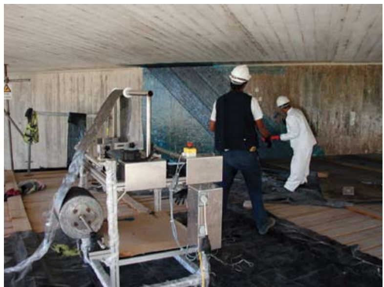
External reinforcement with CRFP fabrics
