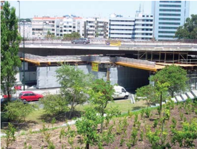
Assembly of the working platform
