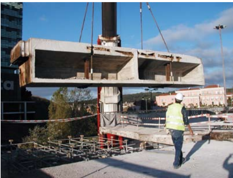
Removal of concrete
