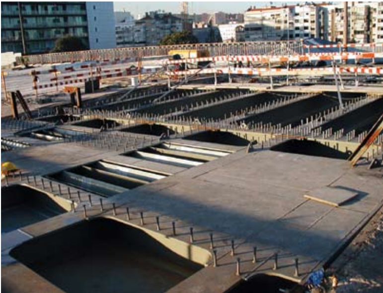
General view of the metal structure
