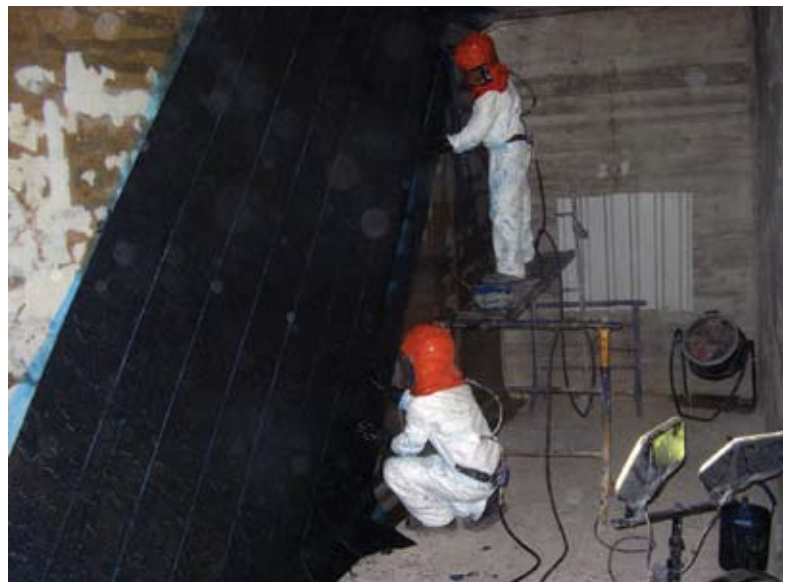
Internal reinforcement with CRFP fabrics
