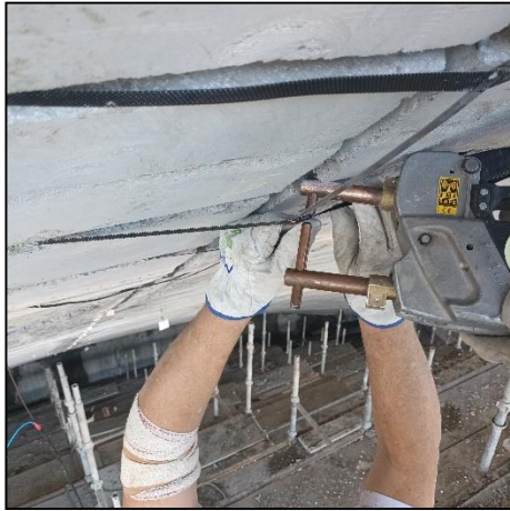
Figure 8 – Spot welding for anode ribbons.
