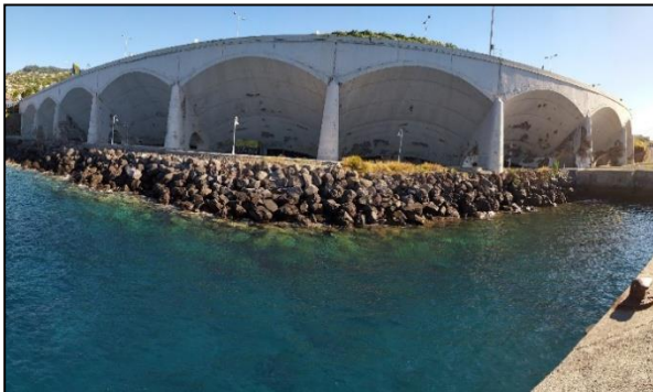
Figure 1 – Front view of the infrastructure.
