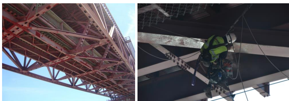
Fig. 6,7 Anti-corrosive coating of the steel rigidity beam.
