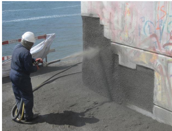
Fig. 14 Concrete repair by sprayed concrete.
