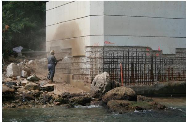
Fig. 13 Sandblasting preparation of damaged concrete surfaces.
