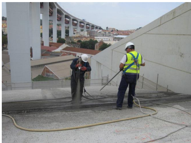
Fig. 24 North anchorage block restoration by sprayed concrete.
