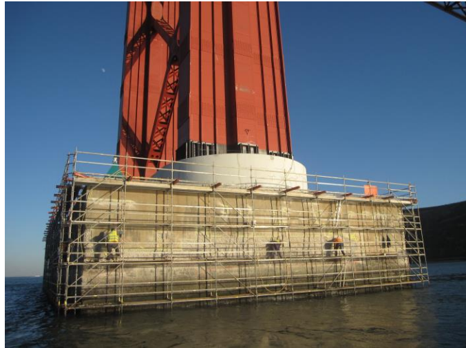
Fig. 9 Scaffolds for the south tower concrete repair works.
