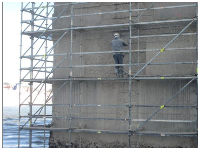
Fig. 10 Sprayed concrete restoration of reinforced concrete.
