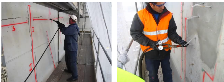
Fig. 25, 26 Treatment of concrete cracks. Concrete injection.
