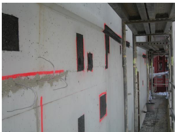
Fig. 19 Hand applied mortar concrete repair and treatment of cracks.
