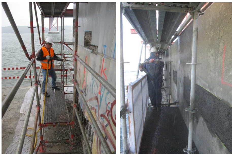
Fig. 11 Preparation of concrete surfaces. Fig. 12 Reconstruction of sections using sprayed concrete.
