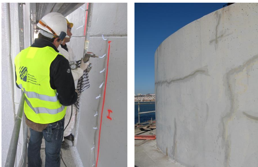
Fig. 17, 18 Concrete injection of cracks.
