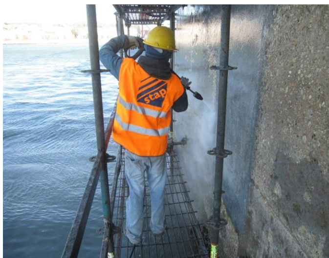
Fig. 20 Preparation of surfaces for the application of final coating system.
